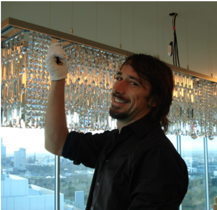
JOHN HOWLAND putting the finishing touches to this 3 metre long Swarovski chandelier. Containing 12,000 Strass Signature Crystal pieces, it weighs 110kgs, and includes a remote controlled RGB LED system creating 16.7 million colours for the ultimate in user friendly customised lighting. Installed in a private residence, Royal Domain Tower, Melbourne, 2007.
